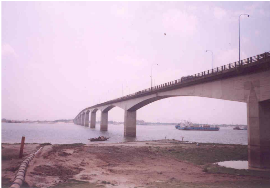
SIDE VIEW OF BRIDGE
