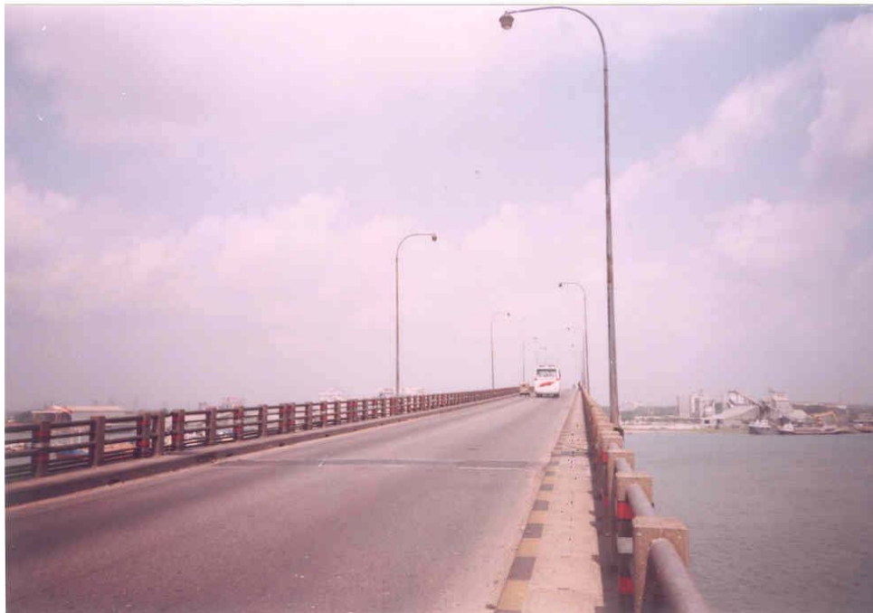
ANOTHER TOP VIEW OF THE BRIDGE
