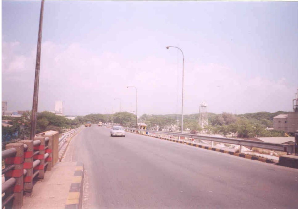
APPROACH ROAD BRIDGE
