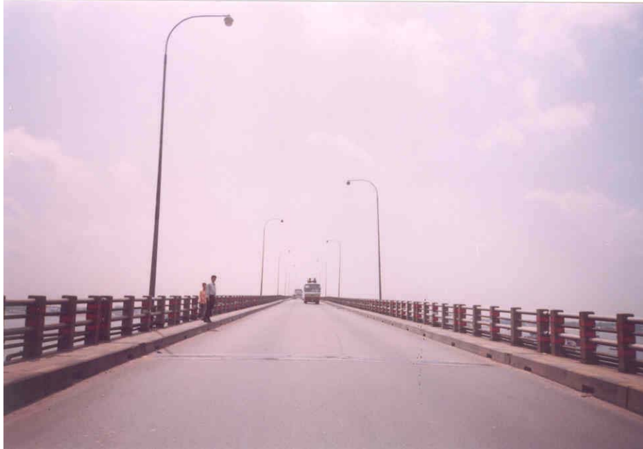
TOP VIEW OF BRIDGE
